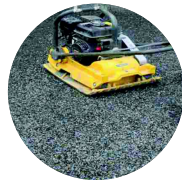
Laying and compaction of leveling layer
