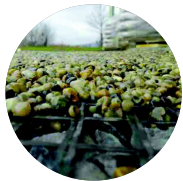
TopStone stone carpet laying
