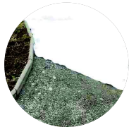
Installation of geotextile
